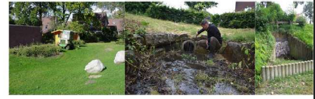
Figure 9.39 From left to right: Mowing swale in Enschede with obstructions, clogged inflow pipe swale in Bee, removal of litter (foul connections) at inlet of the swale in Renkum.
